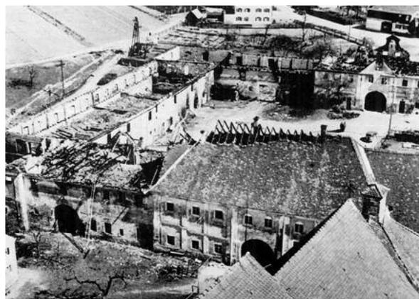
**Bild 6:** Brandbegrenzung durch Brandwände
